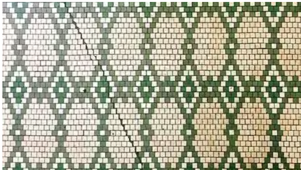
ACCENT TILE AT ELEVATOR LOBBIES & BIKE ROOM
